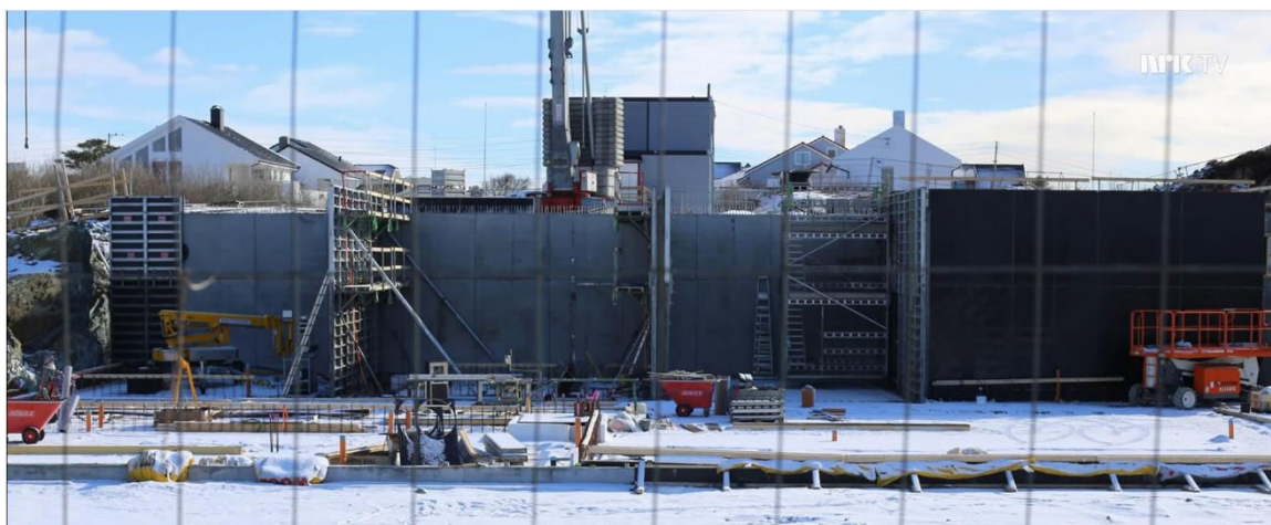
A new primary treatment plant under construction (Photo: NRK).
